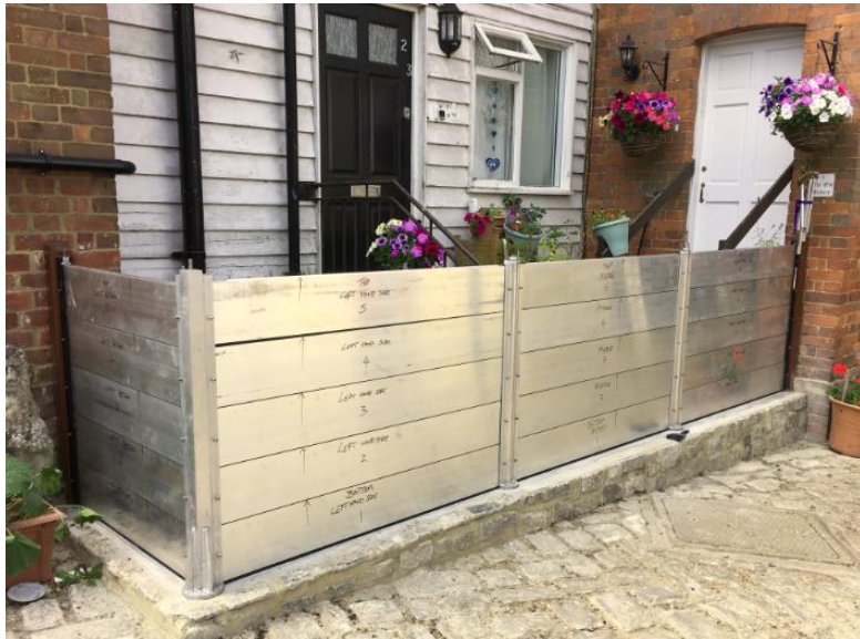
Flood barriers reducing risk to 3 properties
